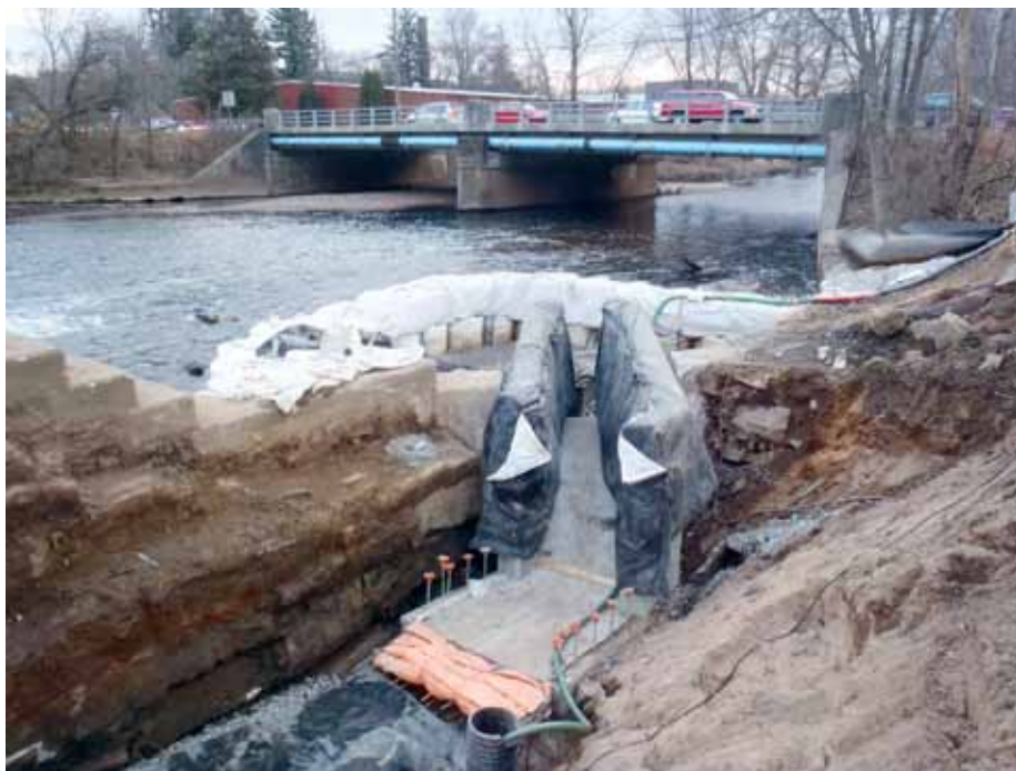
The Wallace Dam Fishway on the Quinnipiac River in Wallingford is currently under construction. The dam is to the left of the photo.
