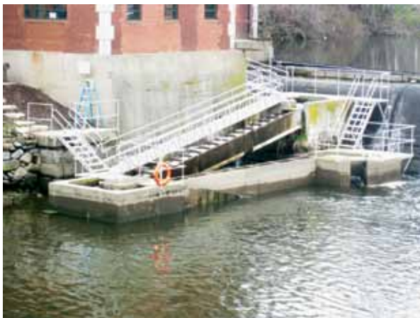
The Mianus Pond Fishway on the Mianus River in Greenwich is a steeppass fishway with two resting pools. It has annually passed 90,000 herring in recent years.
